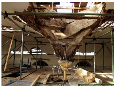
The column under repair
